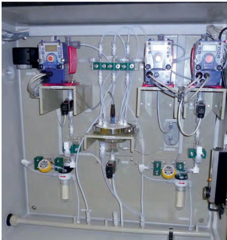
Figure 1: Concentrated hydrochloric acid is diluted 1:3
